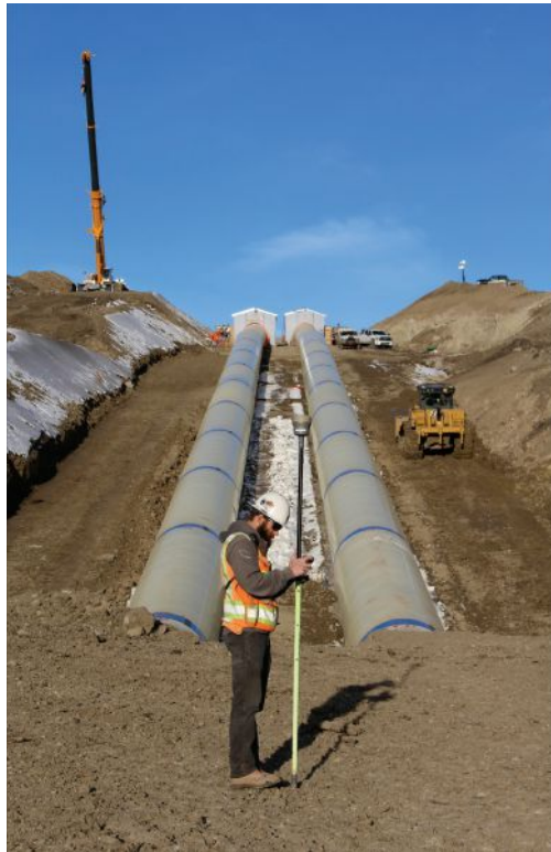
NW CONSTRUCTION SURVEY MANAGER Kenny Neskorik checking backfill.
